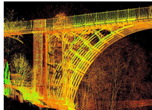
Bridge Lidar Scan
