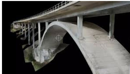
3D Reconstruction of Bridge from Drone Aerial
