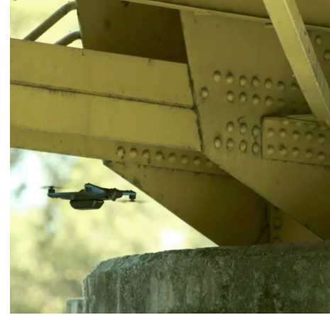
Drone Bridge Inspection
