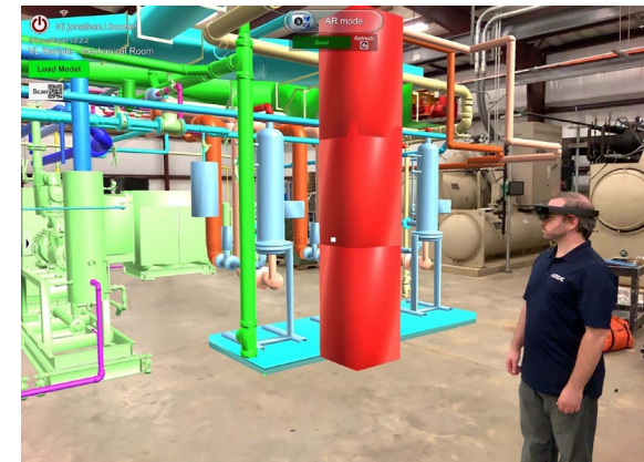
Augmented Reality Facility Management
