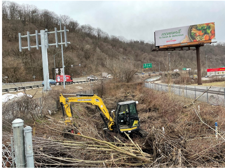
Sediment & vegetation removal
